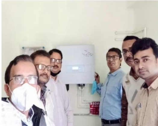
INSTALATION OF SOLAR SYSTEM
