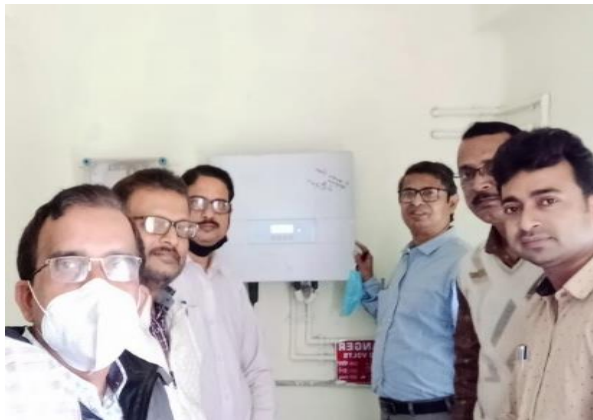
INSTALATION OF SOLAR SYSTEM
